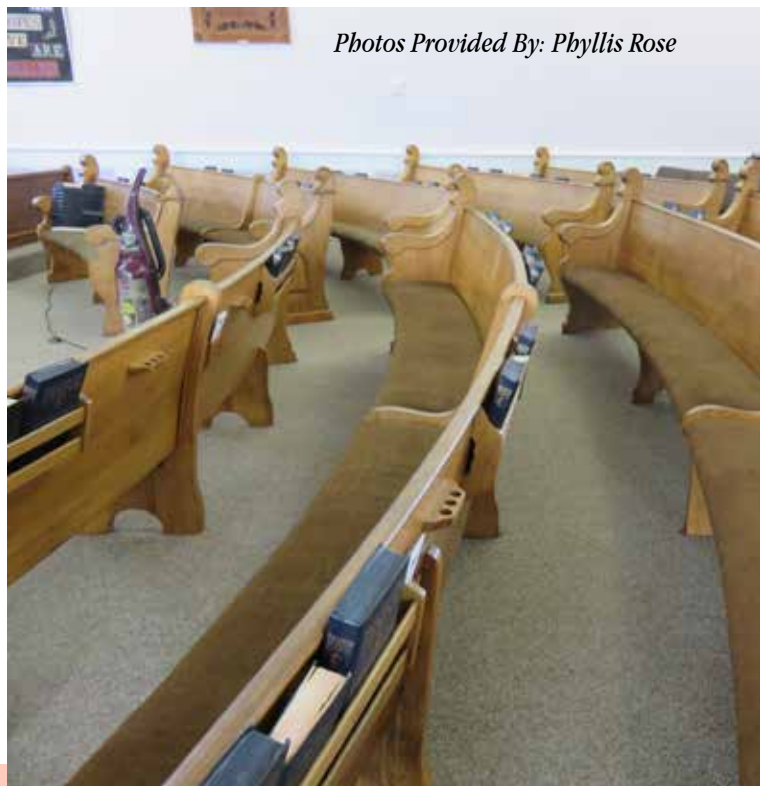
These pews in Mount Zion United Methodist Church are original to the church which was built in 1865.
