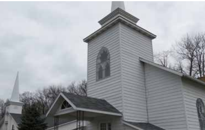
The twin steeples of Clear Lake Bible Church, a church built in 1872 as a Baptist Church.
